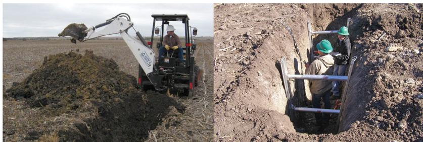
*Left image—A backhoe excavation providing a large view of the soil profile and improving access for description and sampling. Right image—Shoring, exit ramps, and other safety measures must be used to protect staff in deep trenches. (Photos courtesy of Wayne Gabriel)*
